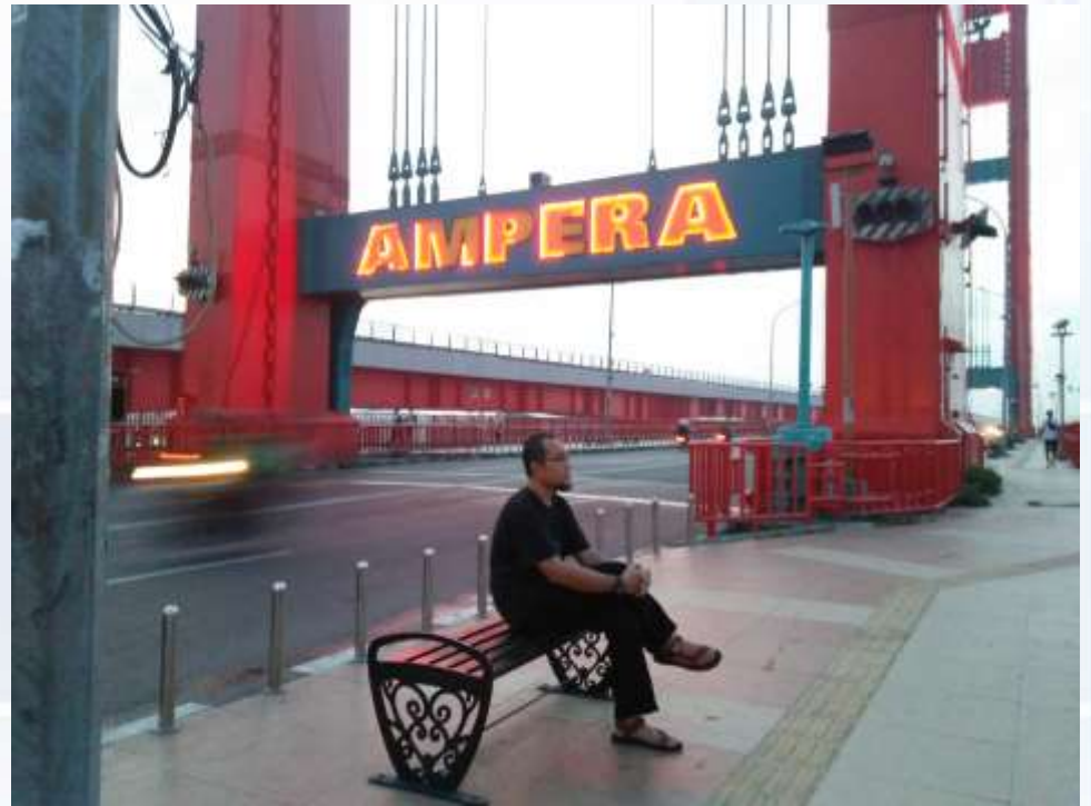
Ampera Bridge, Palembang
